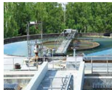
Clarifier Capacity: 660 m 3 /h
