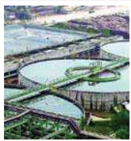
Largest High Rate Clarifier, PT RAPP, Indonesia
