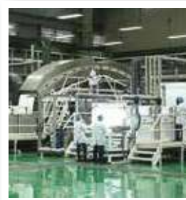
Membrane Manufacturing Unit, Verna, Goa
