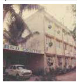
Chemical Manufacturing unit, Ambarnath, Maharashtra
