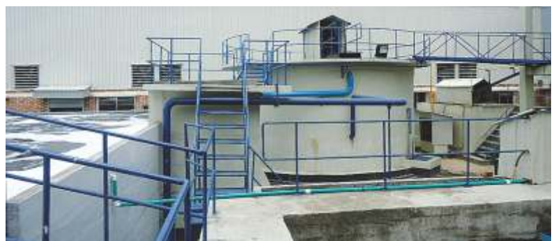
2 x 300,000 USGPD (2 x 1135 m 3 /d) brackish water treatment reverse osmosis plant supplied to Umm Al Quwain, Government of UAE
