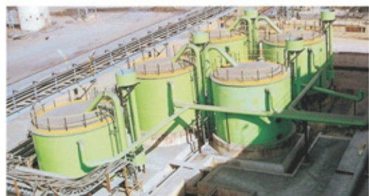
Auto valveless gravity filters
