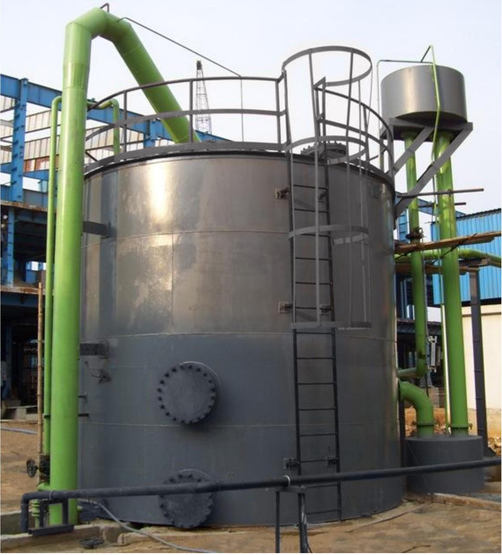
Ion Exchange, pioneer and leader in total water management for over five decades, offers INDION Auto Valveless Gravity Filter (AVGF). The AVGF is a highly efficient automatic filter that operates without any single valve, backwash pump, flow controller or any other instruments. There are no moving parts in the AVGF.
