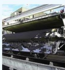
Belt Press for Coal Slurry
