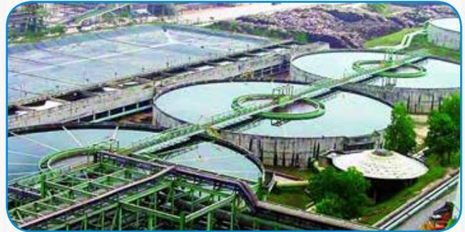
In addition, we supplied DCS controlled chain of demineralization plants with total capacity of 1890 m<sup>3</sup>/h (7 x 270 m<sup>3</sup>/h). This was supplemented by a chain of condensate polishing plants with capacity 1800 m<sup>3</sup>/h (5 x 360 m<sup>3</sup>/h).
