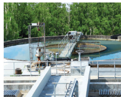
Clarifier Capacity: 660 m 3 /h
