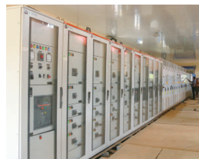
Water Treatment Plant (WTP) pump house main MCC panel (APFC, VFD, AHF)
